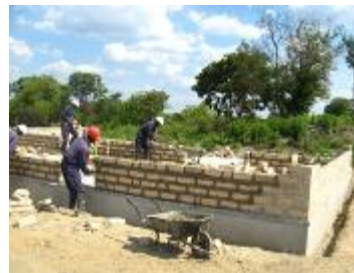
Working on the teacher houses for the High School
