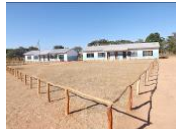
Chibobo Basic School, with a new fence.
